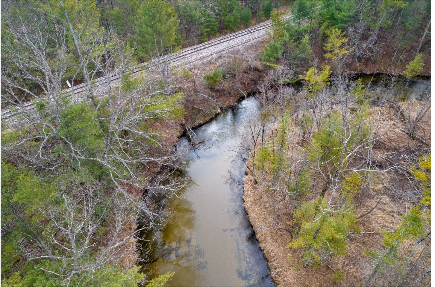
CRA drone photo of the railroad embankment from December 2022.
