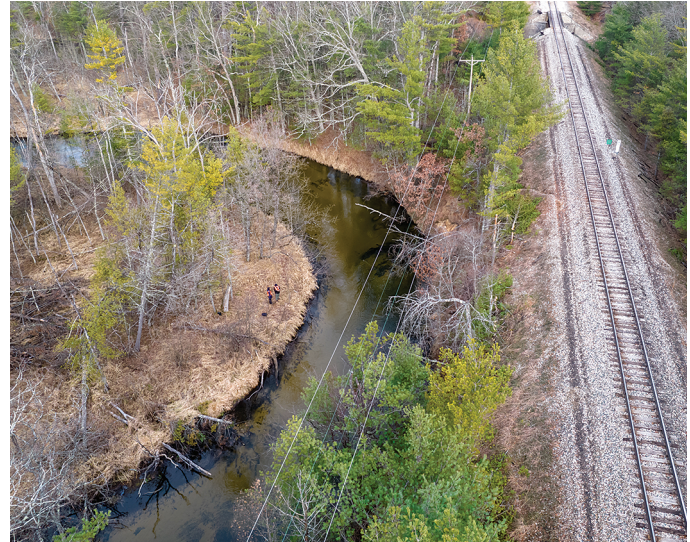
A drone captures the railway atop the embankment as CRA staff investigate the eroding bank on the ground.
