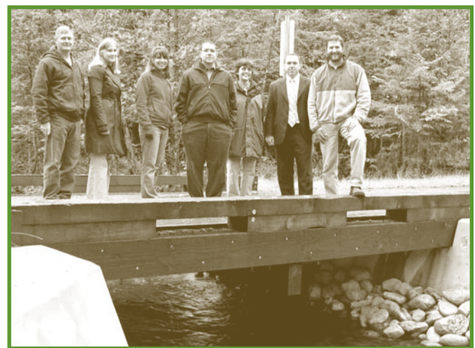
On September 29, 2009 partners celebrated the completion of the Green River Bridge in the Jordan River Watershed. Costs for this timber bridge project totaled $161,500 and included the help and support of 14 different donors and agencies.
