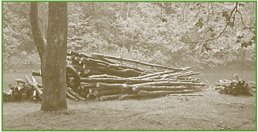
Staging red pines and white oaks to construct fish cover structures.
