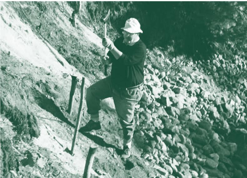
***Big Sable Chairman Jim Miller joined CRA staff in taking the hands-on approach to streambank stabilization. Plans for the eroding bank near Freesoil included rock placement in August, installation of terraces in September and tree planting by the committee in the spring. The stabilization project was funded through a grant from the US Fish and Wildlife Service with matching contributions from the Big Sable Restoration Committee. Thanks for your hard work, Jim!***
