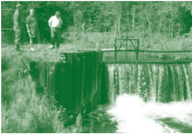
Antrim County's Green River Dam prevents upstream and downstream migration of fish.
