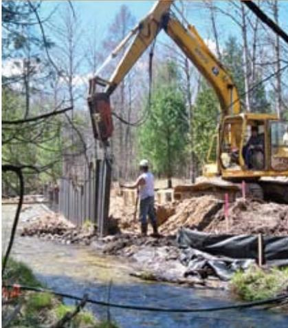
The McDowell Construction crew drive sheet piling for the new crossing structure.
