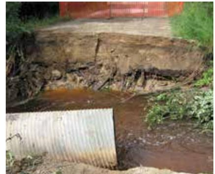
Above - An undersized culvert contributed to road failure during a heavy rain event. Below - A newly installed crossing benefits the entire watershed.
