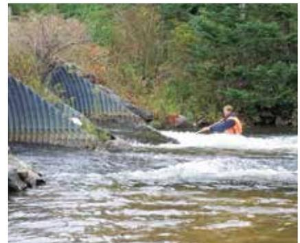
Stream velocities at the outlet of the culverts exceed 5 times the velocity measured on the Jordan River upstream and outside of the impacted area.
