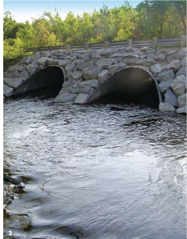
1. Before – exposed embankments and foot traffic were problems. 2. Rock was strategically placed to allow recreational access. 3. After – large, heavy rock protects the embankments.
