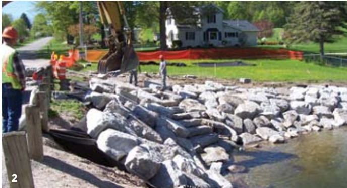
1. Before – exposed embankments and foot traffic were problems. 2. Rock was strategically placed to allow recreational access. 3. After – large, heavy rock protects the embankments.
