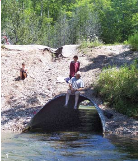
1. Old culvert fill constantly eroded and washed into the Platte. 2. Bridges are ideal for mainstem crossings, allowing the river to flow freely under the road.
