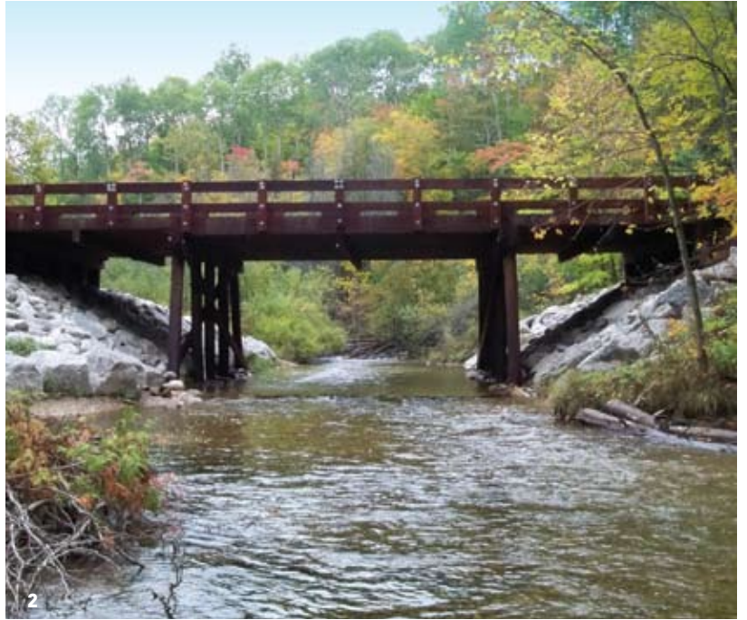
1. Old culvert fill constantly eroded and washed into the Platte. 2. Bridges are ideal for mainstem crossings, allowing the river to flow freely under the road.
