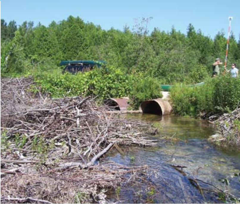
1. Before – frequent beaver activity required maintenance. 2. The road constantly washed into the stream. 3. After – a timber bridge provides access to recreationists and allows for a natural stream bottom.
