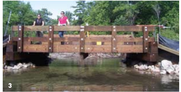
1. Before – frequent beaver activity required maintenance. 2. The road constantly washed into the stream. 3. After – a timber bridge provides access to recreationists and allows for a natural stream bottom.
