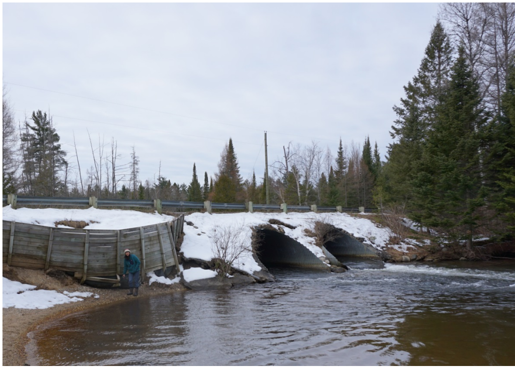
Caption: The current double 16' wide culverts that sit where Old State Road crosses the Jordan River are slated for removal this spring.
