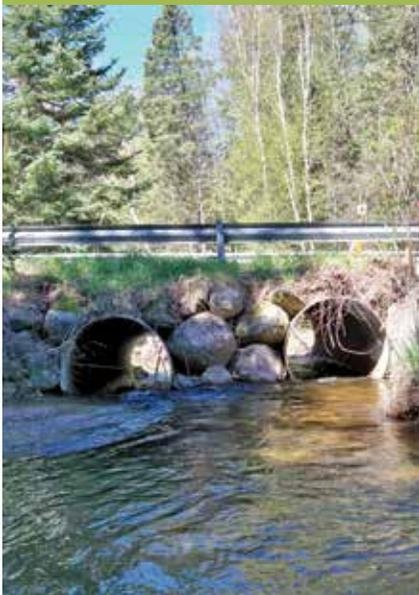
Undersized, perched culverts at Springbrook Road on the main-stem of the North Branch of the Boyne River will be replaced with a timber bridge thanks to support from the US Fish & Wildlife Service, Oleson Foundation, and the Charlevoix County Community Foundation.
