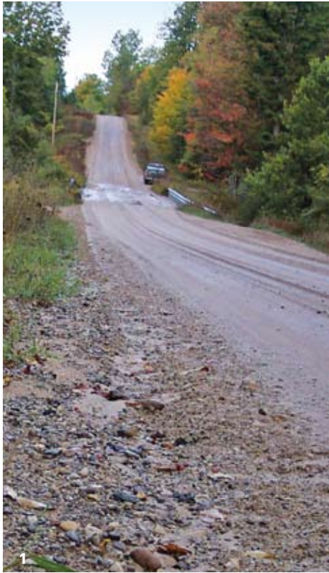
1. Before - sand and gravel repeatedly washed down the approaches. 2. During construction. 3. Spillways handle runoff and filter out sediment. 4. After - pavement is the only effective solution.
