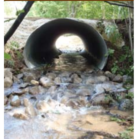
Now there is a properly sized and installed new culvert.
